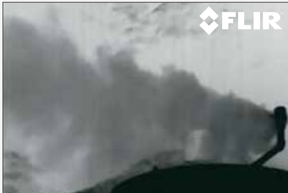
Venting storage tank pressure relief valve.
