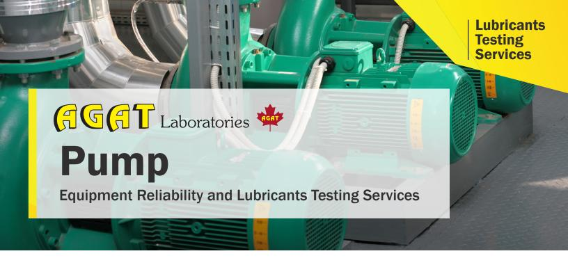
Industrial pumps come in all designs; positive displacement pumps may be reciprocating (piston, plunger, or diaphragm), or rotary (gear, screw, lobed or vane design). Centrifugal pumps are either axial or radial in design and the latter may be mounted vertically or horizontally.
